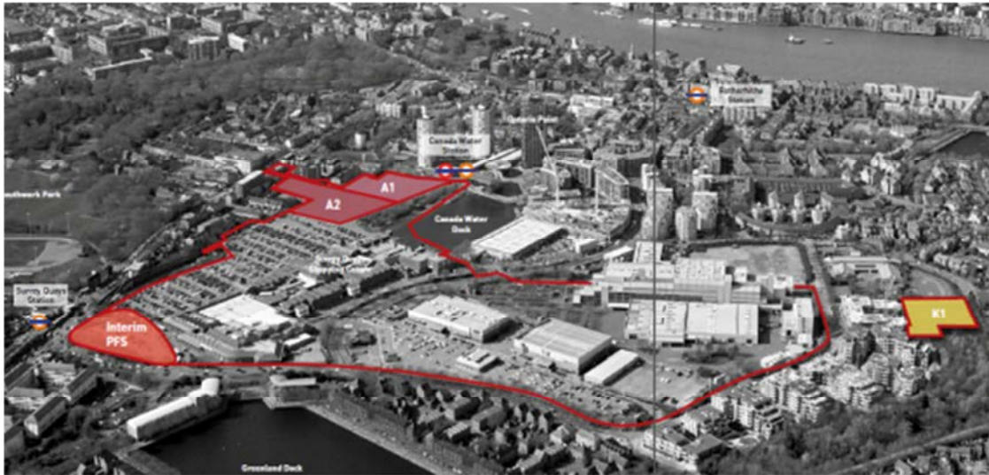
Figure 2: Aerial Photograph of site identifying Detailed Plots
