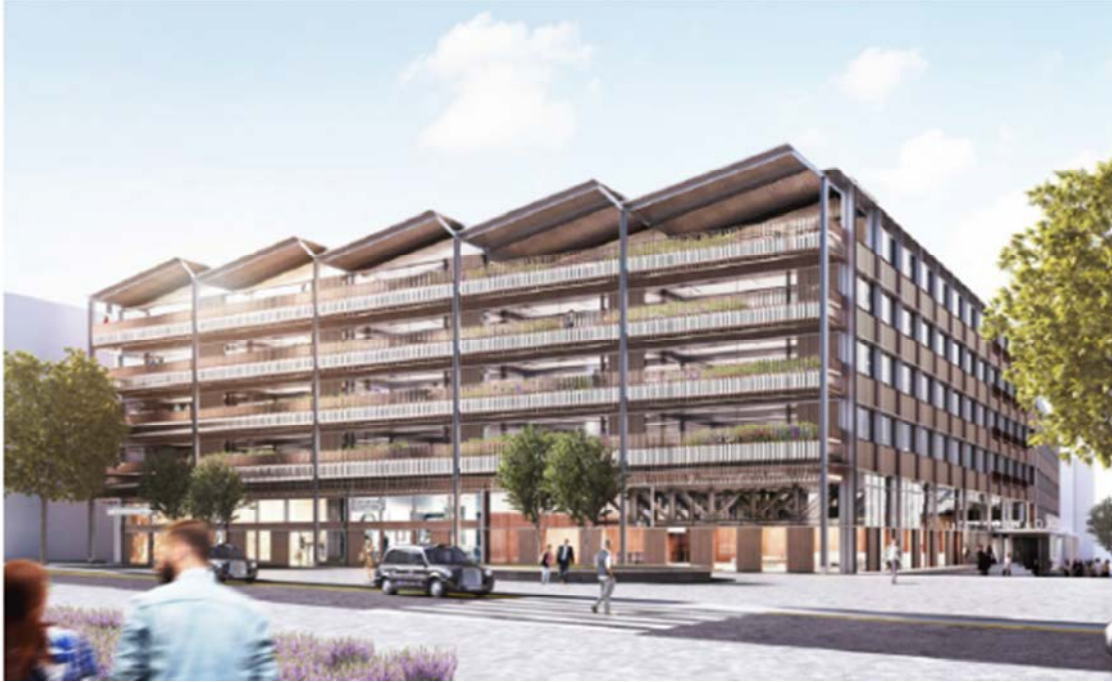
Figure 4: A2 building viewed from the southern edge of Canada Water Dock
